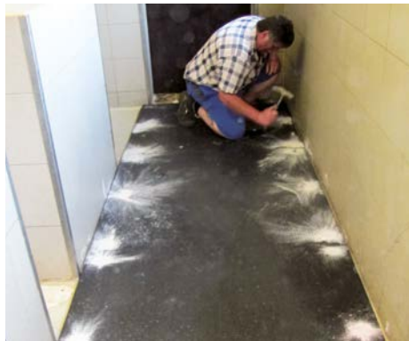
then the mats are fastened with nail plugs
