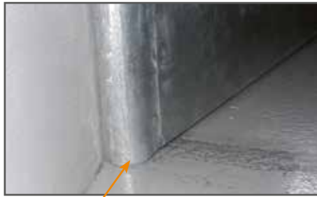
side cleaning flap attention: sharp edges! (-> round off!)
