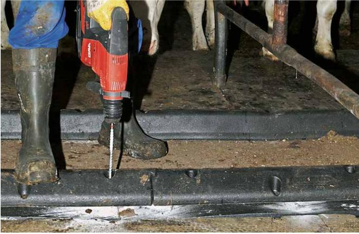
The solid rubber cleats are 175 cm long and 11 cm high. For installation holes have to be drilled into the floor every 35 cm. Afterwards they are fastened, so that the first centimetres of the rubber mats are overlapped.
