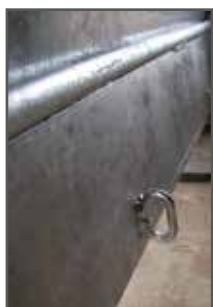
chain links welded on
